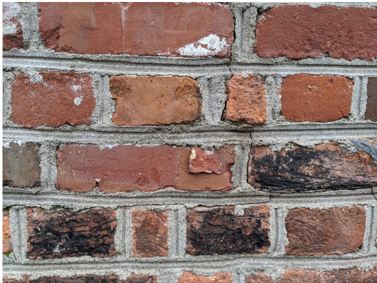
Figure 15 - Cracks along the brick/mortar interface
