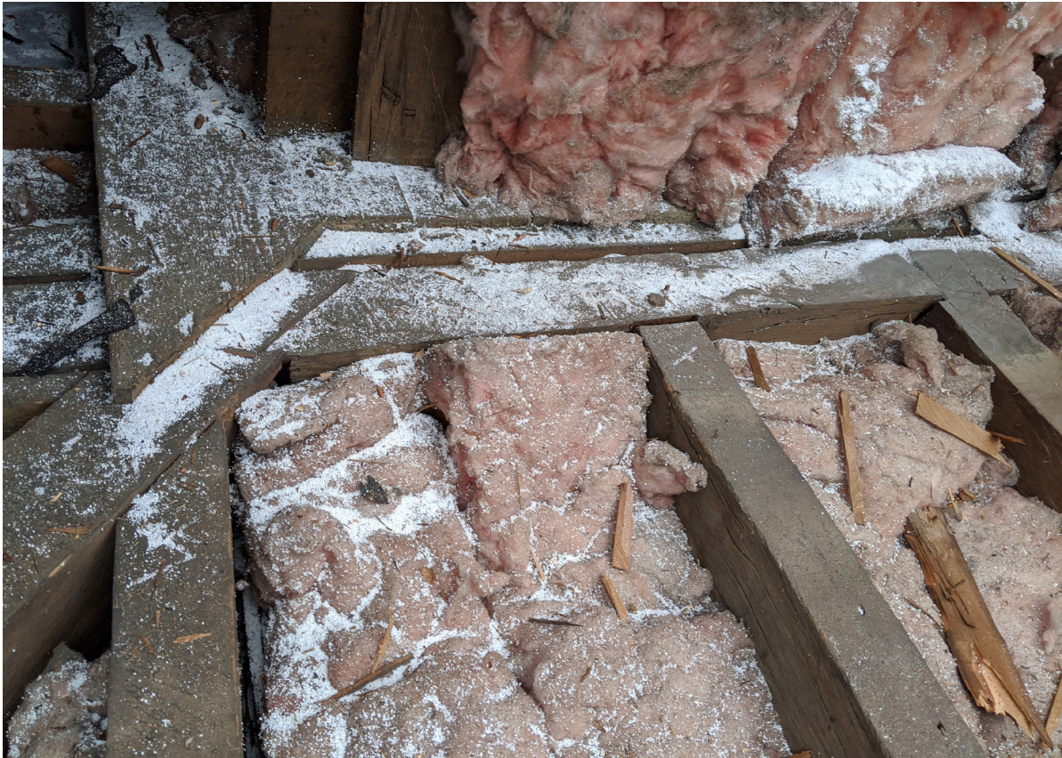
Figure 27 - As-found conditions of 3rd floor ceiling joists to outlooker.
