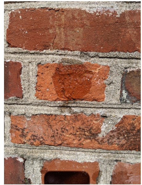
Figure 14 - RILEM test location on brick face without fireskin on northwest chimney
