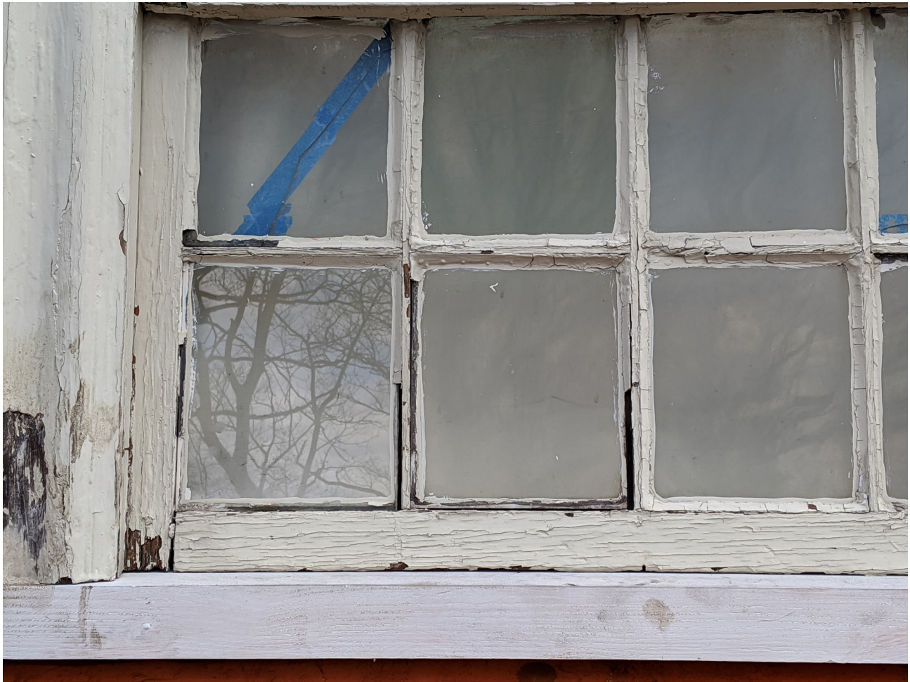
Figure 35 - Failing paint and glazing on east window of SW elevation
