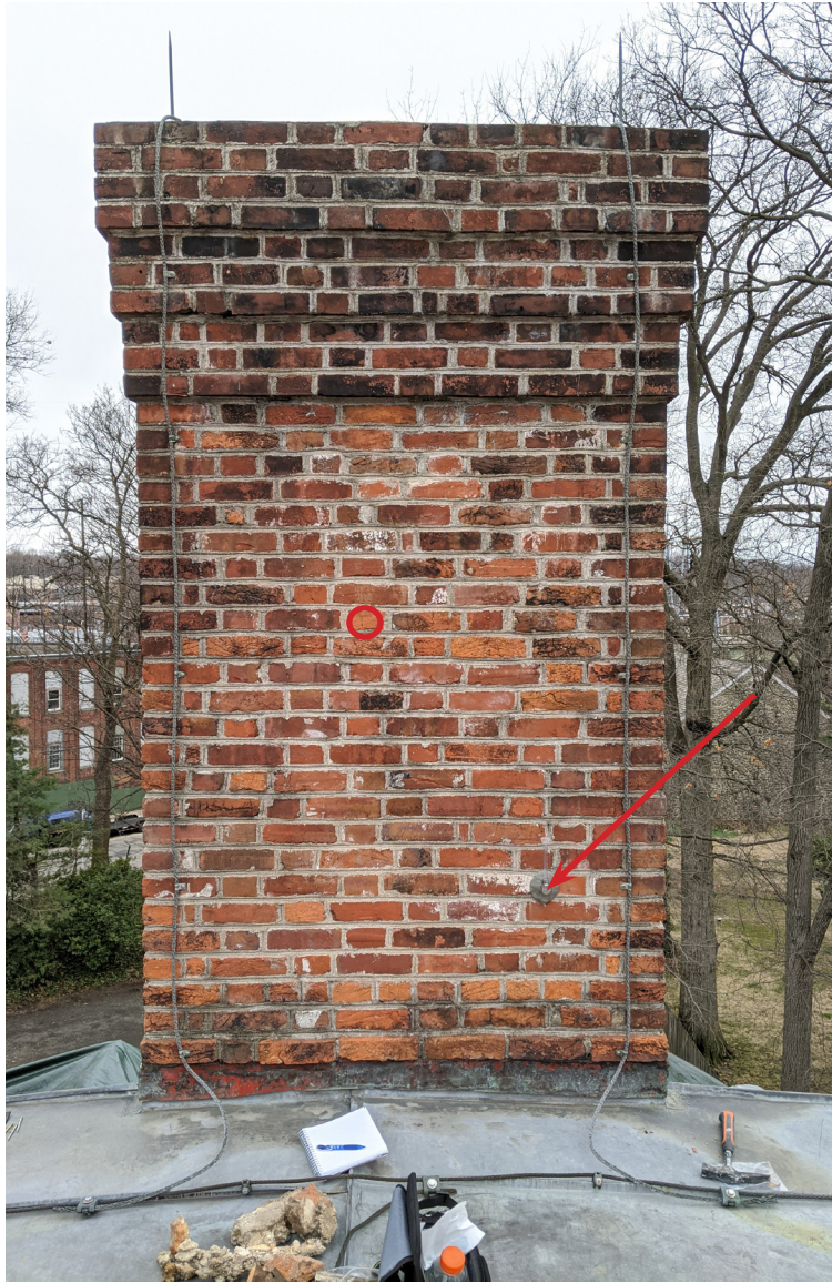
Figure 7 - Northwest chimney with RILEM test location on a mortar joint called out by red arrow and test location on a brick face called out by a red circle
