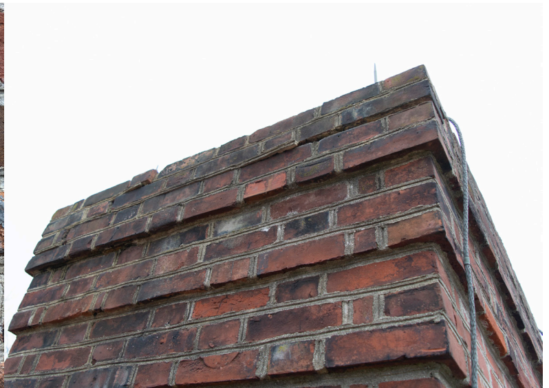
Figure 16 - Mortar moving away from joints, creating open joints allowing water infiltration
