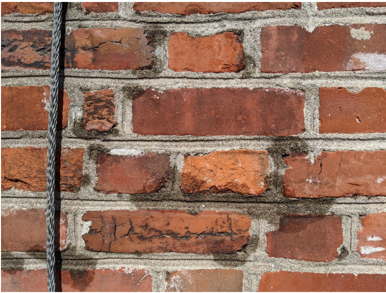
Figure 13 - Water movement through cracks along the mortar/brick interface to evaporate on the warm surface.
