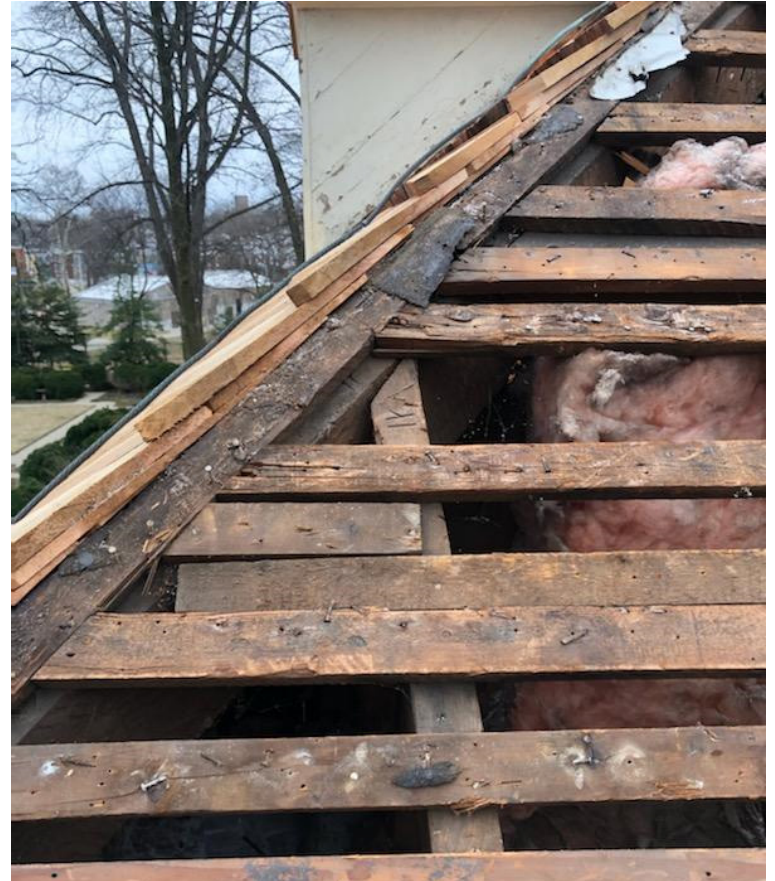
Figure 40 - Marriage mark visible on rafter. Location 1 on subsequent drawing.
