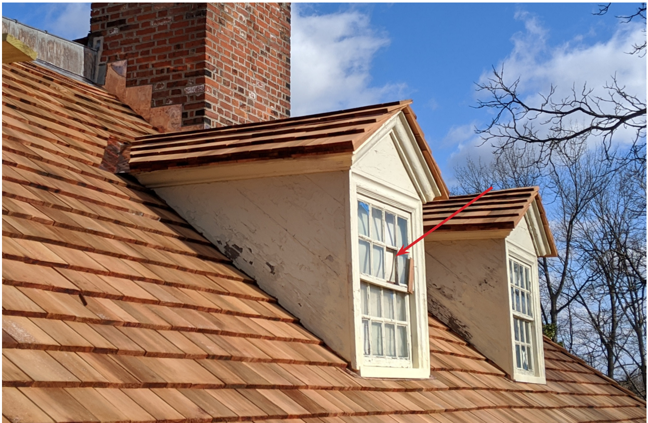
Figure 36 - Missing pane of glass on SE elevation indicated by red arrow
