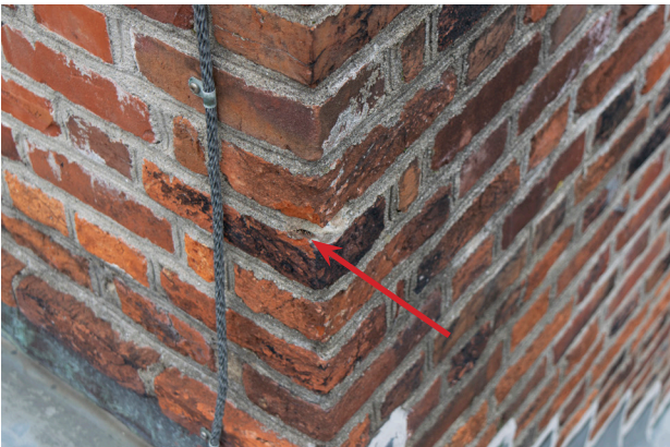
Figure 3 - Sampling area on southeast chimney called out with red arrow
